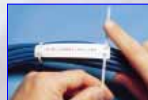
Attach marker to cable with Panduit cable ties
